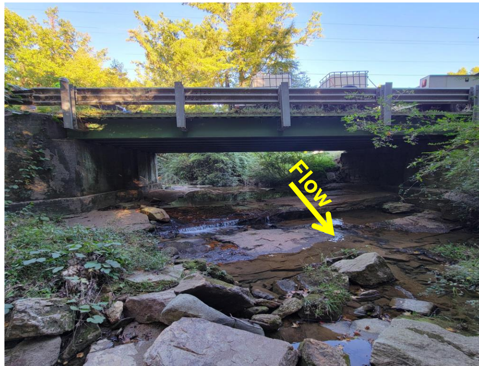
View of Bridge 235 over Beaver Creek looking northwest.
