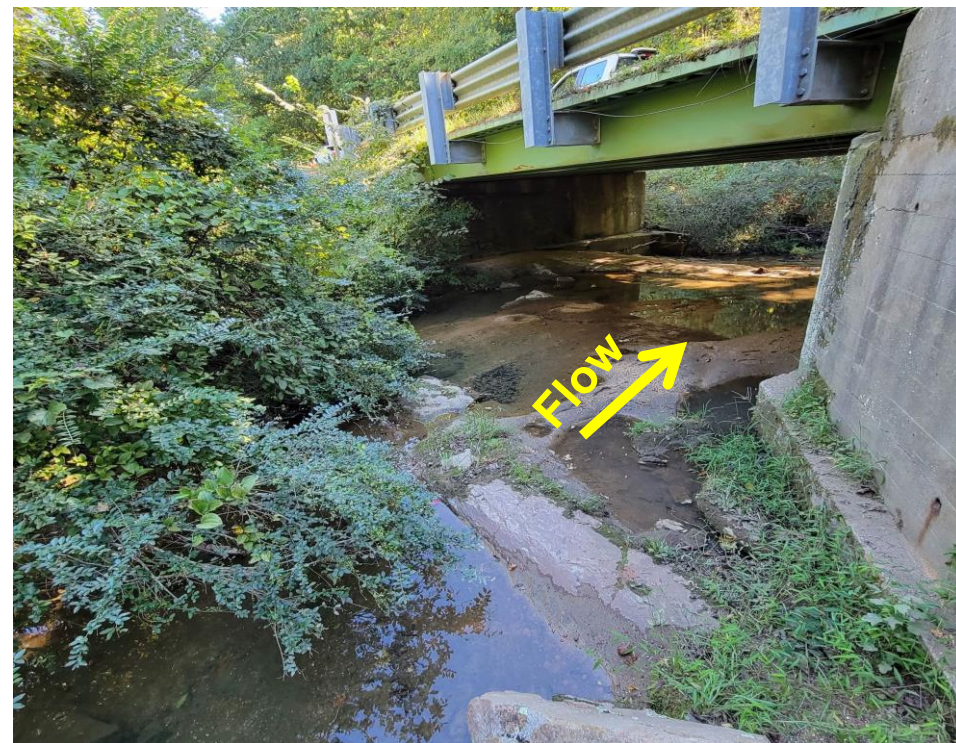
View of Bridge 235 over Beaver Creek looking east.
