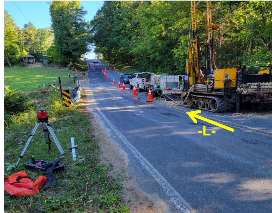
View of SR 1322 looking northeast.
