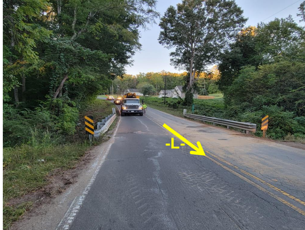
View of SR 1322 looking southwest.
